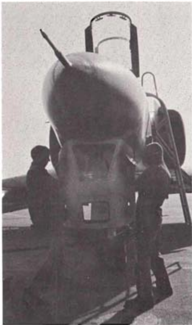
Loading an RF-4 reconnaissance jet with film.
